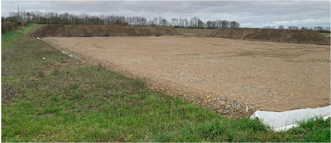
Photo 15.15: Newly Installed Construction Compound
