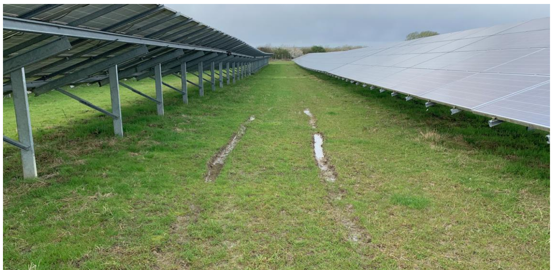
Photo 15.21: Example of Minor Ruts Caused by Vehicles
