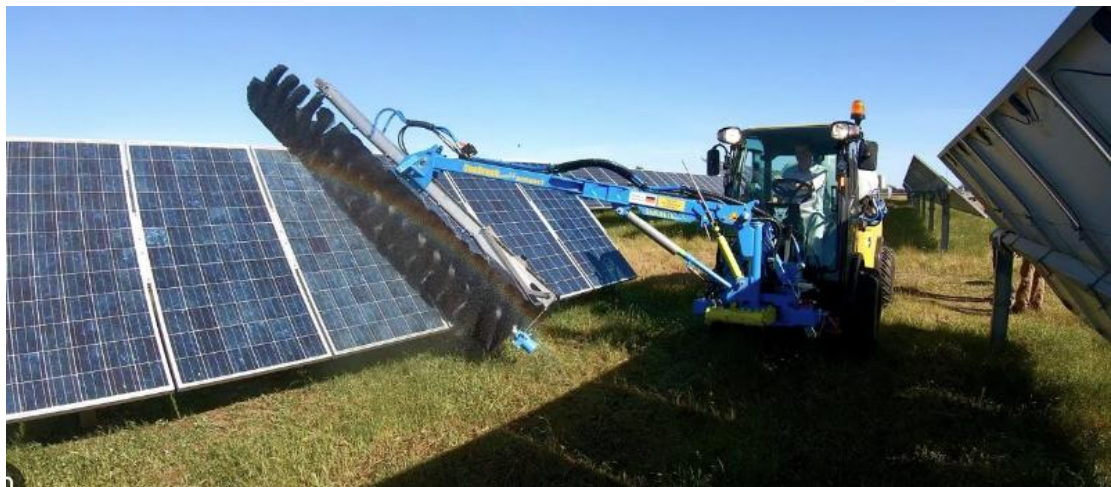
Photo 15.20: Cleaning of Solar Modules
